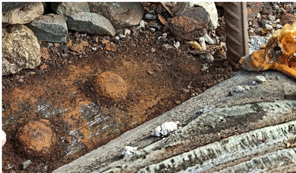
Obr. 3.36. Stav horní plochy na žlabinách Fig. 3.36 Condition of the upper surface on the gutters
