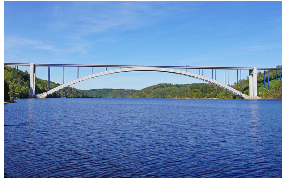
Fig. 3.155 View of the bridge from the west in 2020
