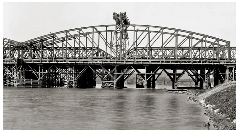
Fig. 1.1 (a, b) Railway bridge under Vyšehrad
