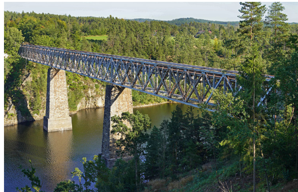
Fig. 3.1 View of the bridge from the northwest
