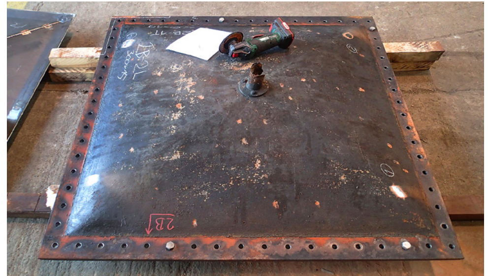
Obr. 3.15. Pohled na demontovanou puklovku Fig. 3.15 View of the removed buckle plate
