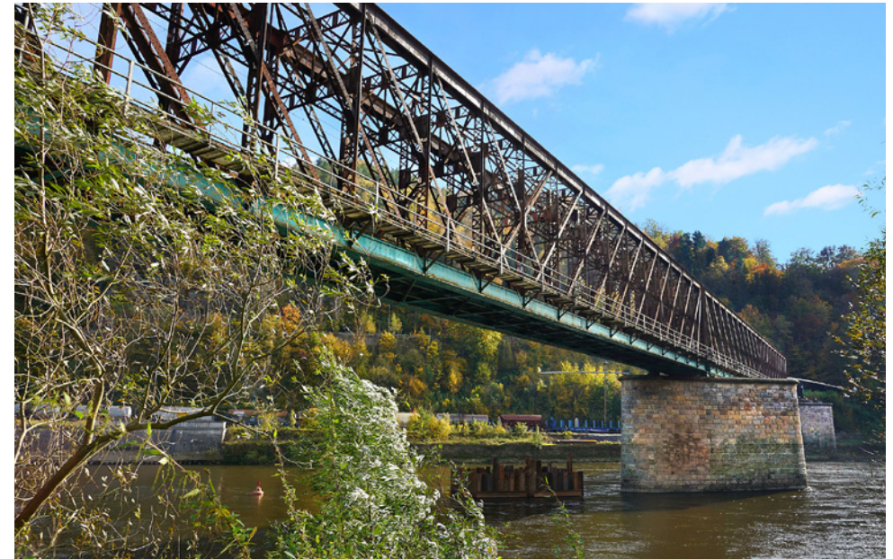
Fig. 3.39 View of the bridge from the west in 2020
