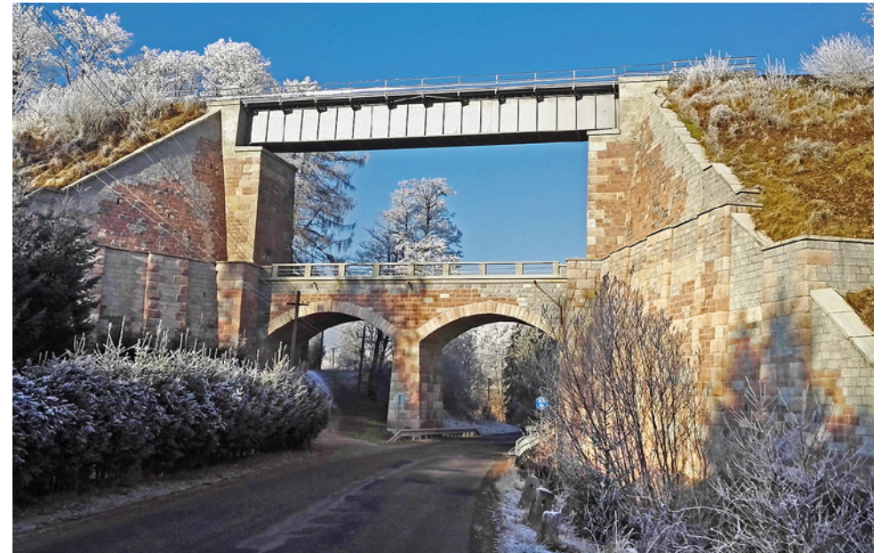
Fig. 3.47 View of the bridge from the south-east in 2019 (photo: authors' archives)
