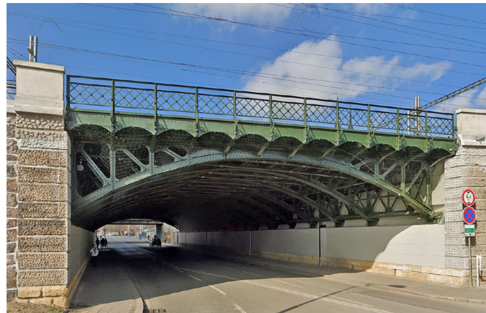
Fig. 3.10 View of the bridge from the south in 2021
