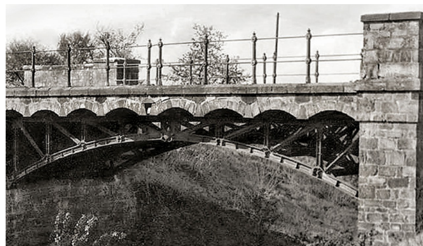
Fig. 1.5 Cast iron bridge near Nemilany (a) and Hoštěrádky-Řešov (b)
