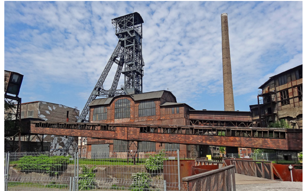
Fig. 3.176 View of the conveyor bridge in 2018
