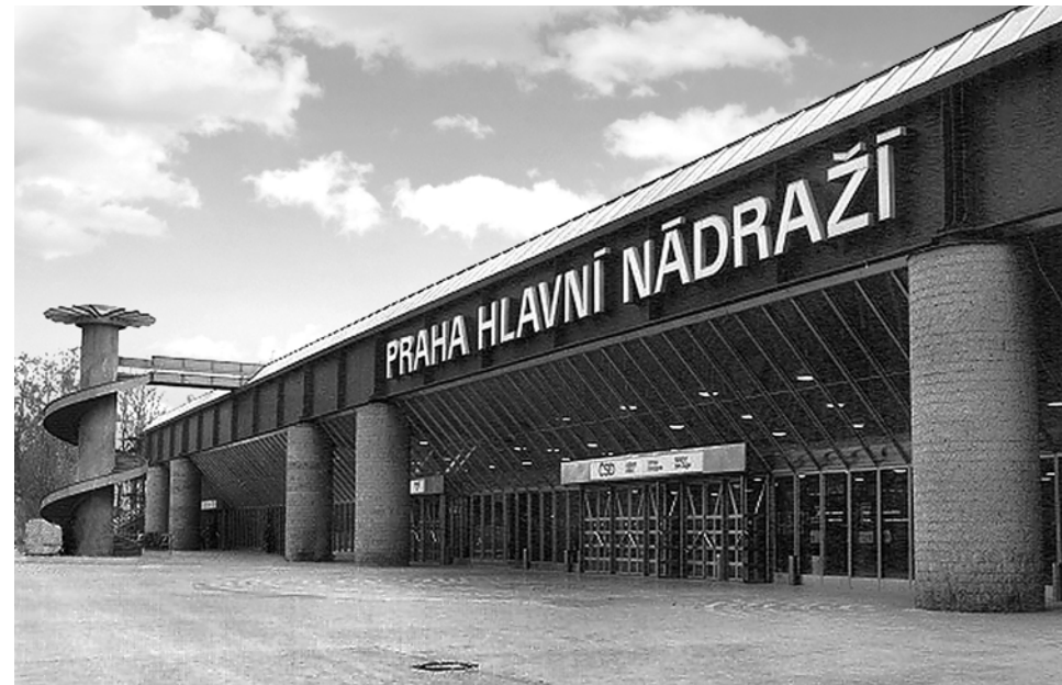
Fig. 1.45 Prague Main Railway Station; (a) spiral staircase after hot spraying in 1977, (b) finalized station
