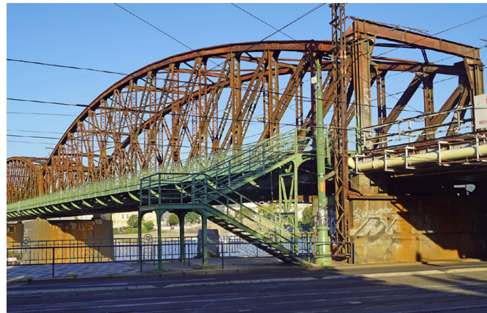
Fig. 3.20 View of the bridge from the southeast in 2021
