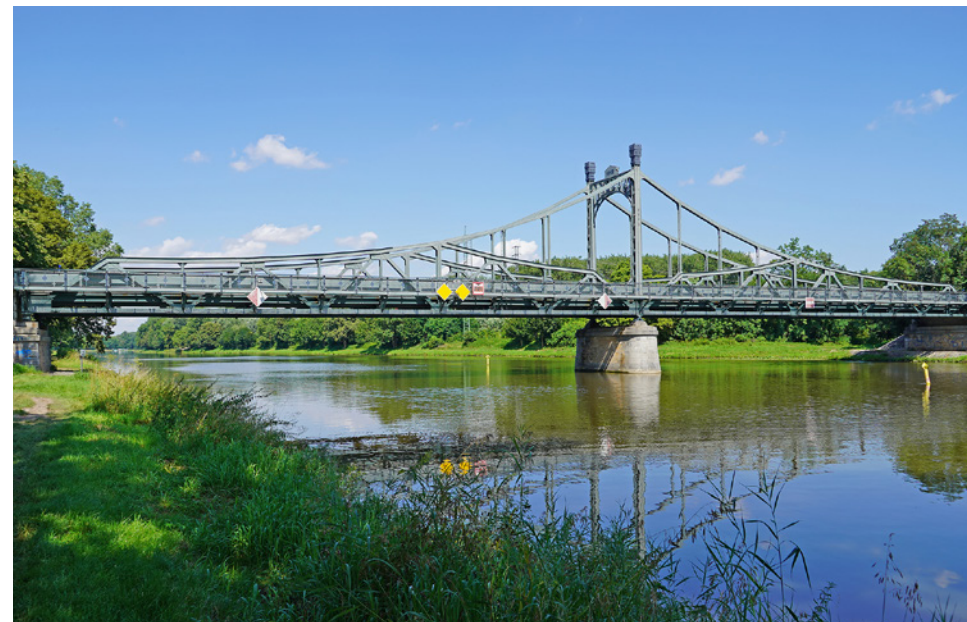
Fig. 3.112 View of the bridge from the west in 2020
