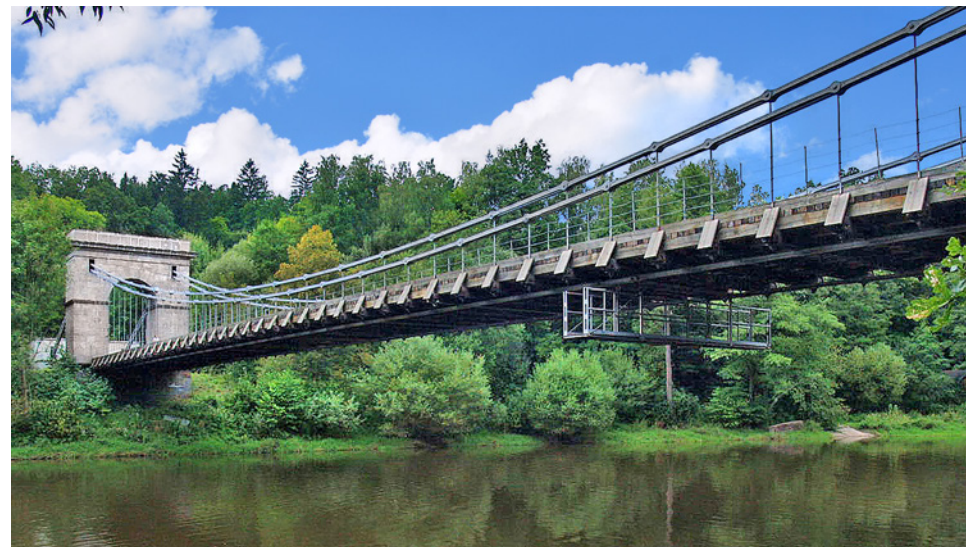
Fig. 1.2 (a, b) Suspension bridge in Stádlce
