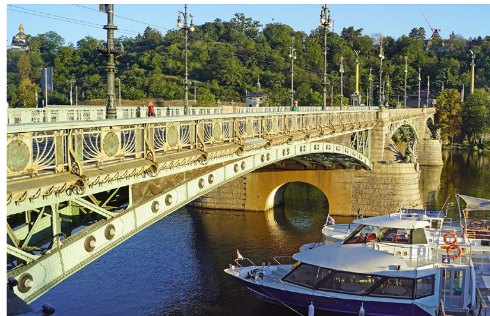
Fig. 3.103 View of the bridge from the west in 2020
