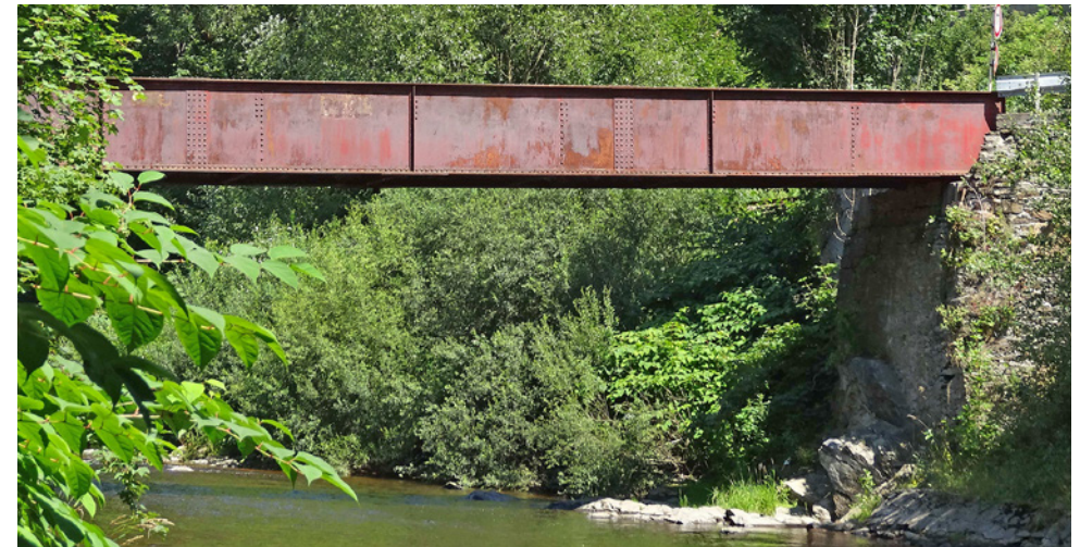
Fig. 3.68 View of the bridge from the south in 2020
