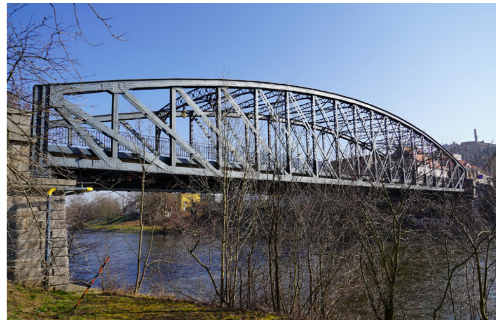
Fig. 3.83 View of the bridge from the west in 2020
