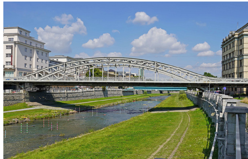
Fig. 3.123 View of the bridge from the southeast in 2021
