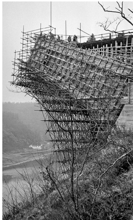
Obr. 3.157. Stavba mostu 1957–1960 Fig. 3.157 Construction of the bridge 1957–1960
