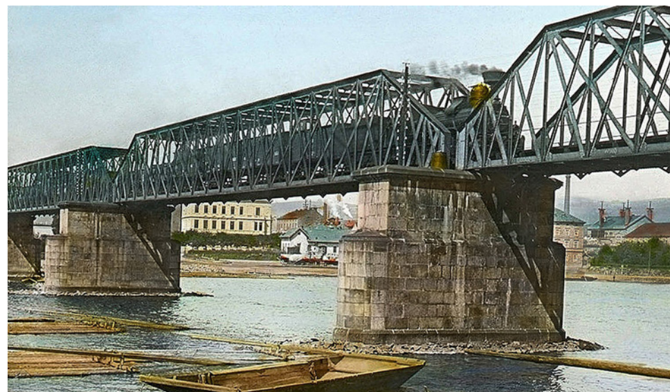
Fig. 1.24 (a, b) Truss half-through bridge with straight chords (railway bridge in Prague under Vyšehrad from 1871)
