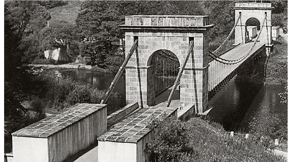
Fig. 3.59 (a, b) Original position of the bridge in Podolsko
