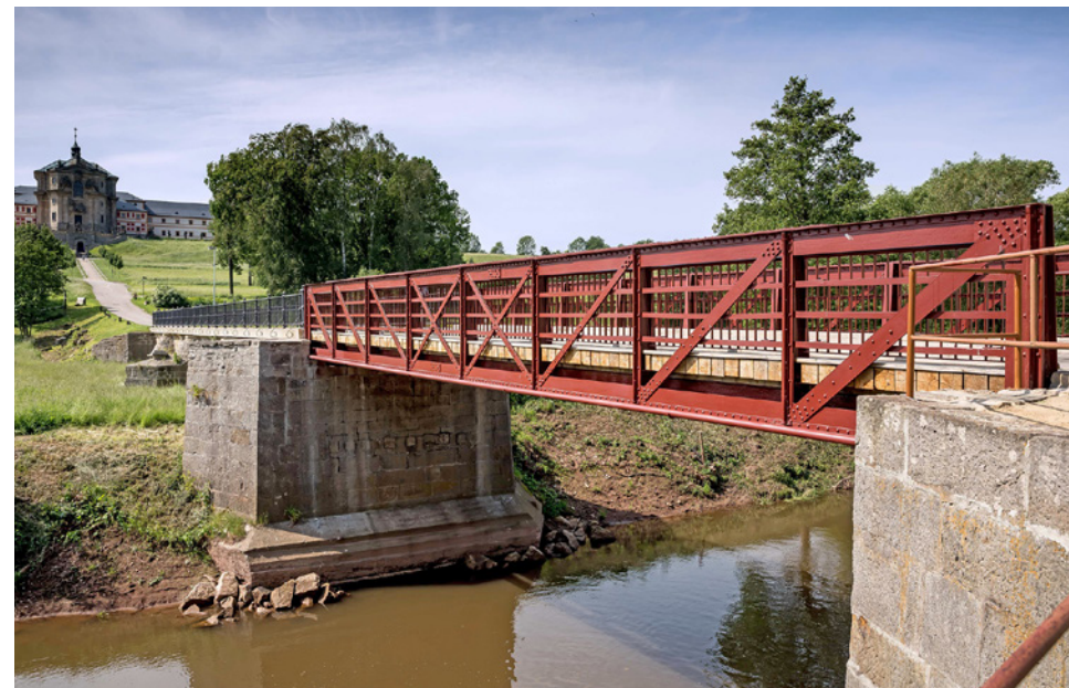
Fig. 3.77 View of the bridge from the northeast in 2021 (photo: authors' archives)
