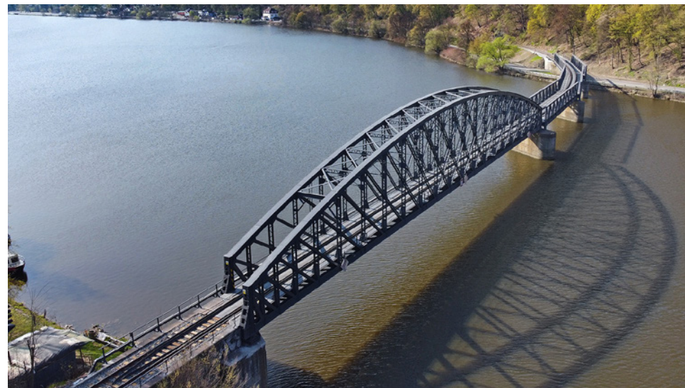
Fig. 1.4 (a, b) Bridge in Skochovice
