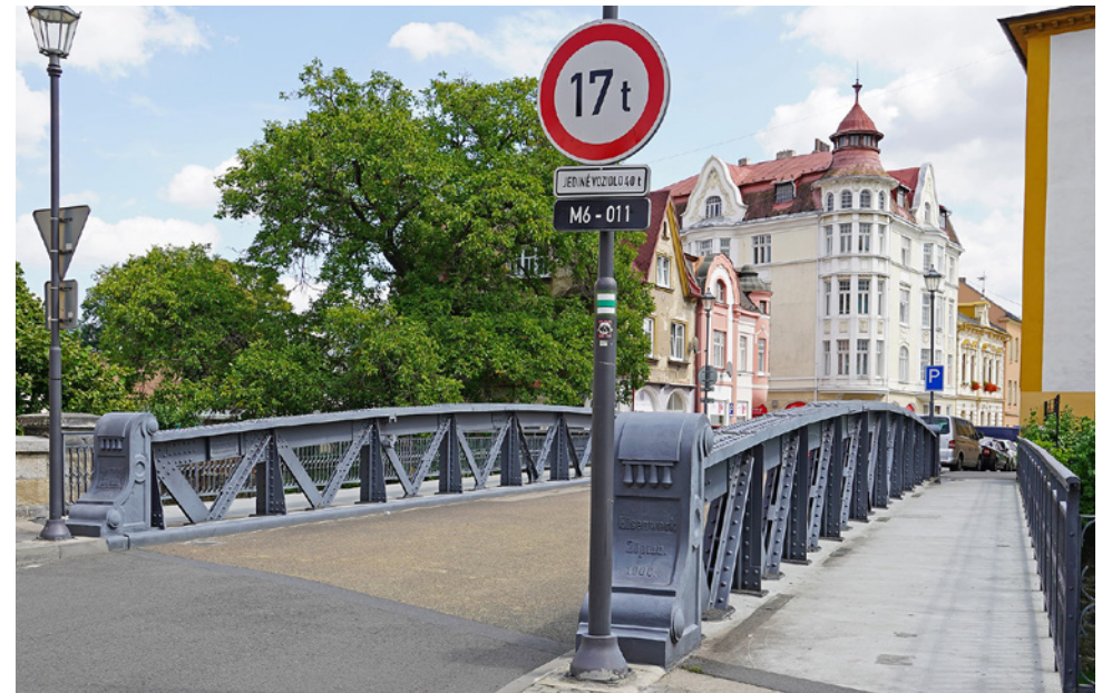
Fig. 3.92 View of the bridge from the west in 2019
