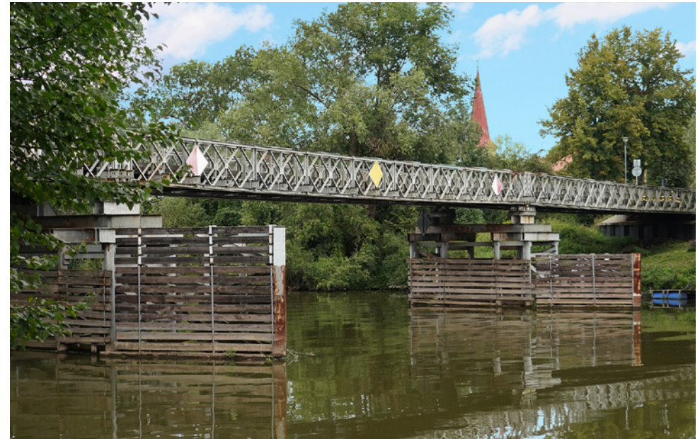
Fig. 3.146 View of the bridge from the east in 2021
